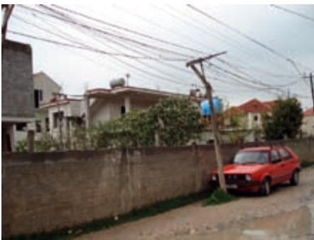
Figure 2c: Illegal connections in Albania. (Source: private collection D. Andoni)
