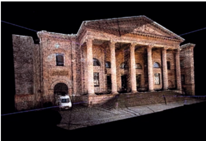
Figure 22: Results of a terrestrial scanning of a complex facade.
