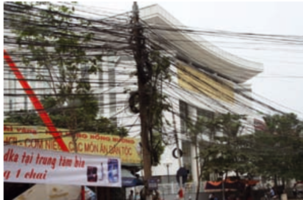
Figure 2b: Energy supply infrastructure, Hanoi. (Source: private collection C. Potsiou, 2009)
