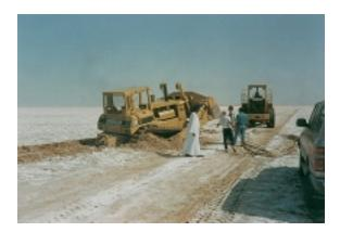
Fig 7: Establishment of a new track facing problems with salt lakes
