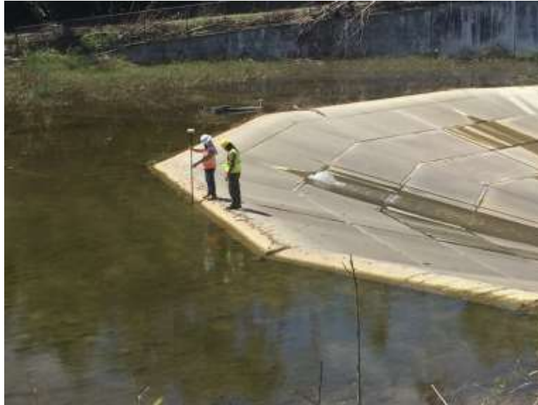
Figure 10. Land Surveyors perform As-built Survey applying Real-Time Kinematic (RTK) techniques at Guajataca Dam after hurricane Maria. (Seda, 2017)
