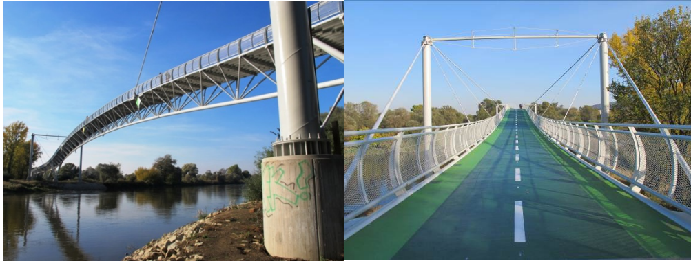
Fig. 3 Liberty cycling bridge
