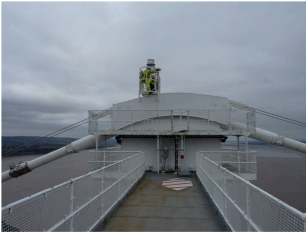
Figure 4. The GNSS antennas located at survey point T2 on the Bridge, the north side Beachley end. The illustration shows the choke ring GNSS antenna being installed.
