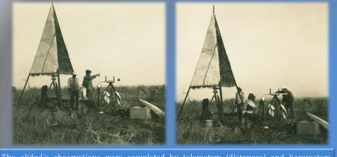
The alidad's observations were completed by telemeters (distances) and barometers (heights) measurements. The toponymy was collected in the villages.
