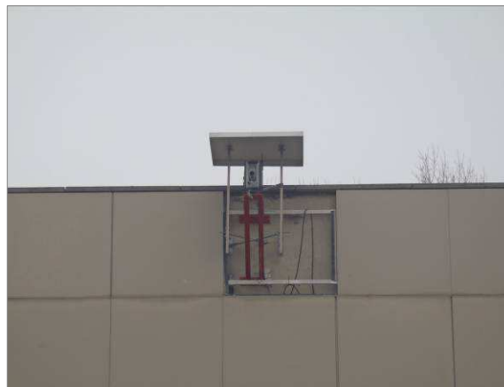
Figure 4: Installation of a Trimble S8 total station on site
