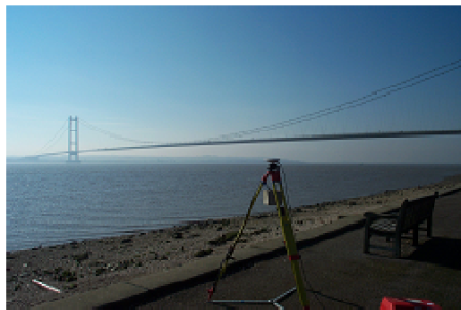
Figure 5. The Humber Bridge showing a GPS receiver reference station in the foreground
