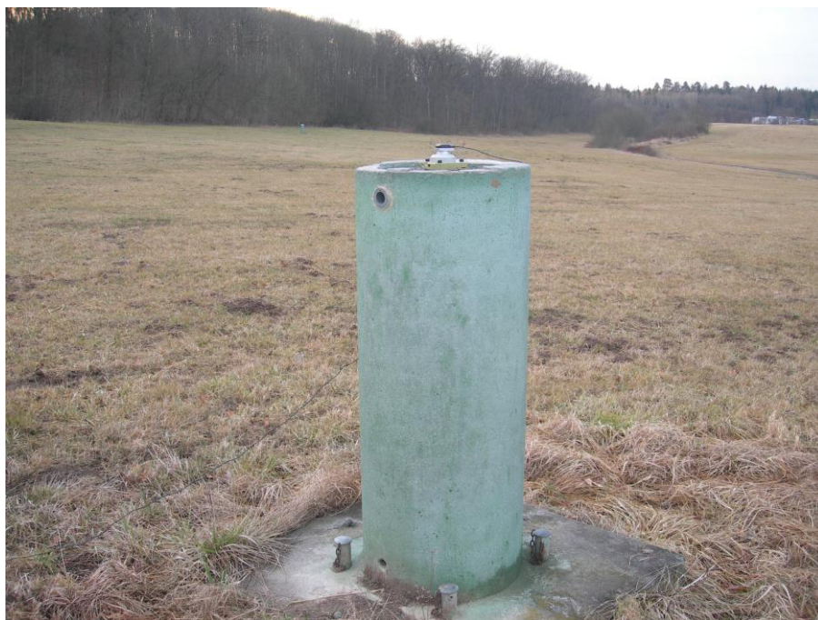
Figure 8: u-blox receiver within IAGB pillar network
