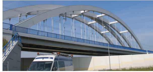
Figure 2. View of the tested bridge
