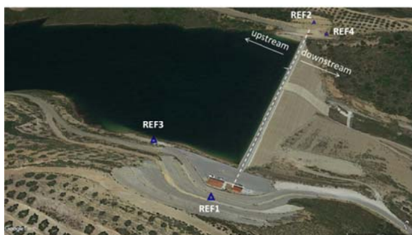
Figure 2: Location of reference pillars for monitoring in “Valsamiotis” dam.
