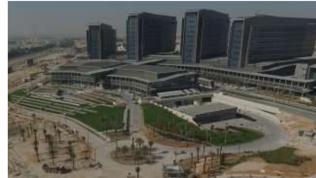
Hospital in Abu Dhabi
