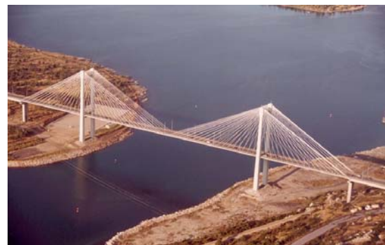
Figure 3. Evripos cable-stayed bridge
