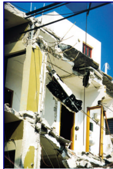
7 b . Partial collapse of the load bearing system
