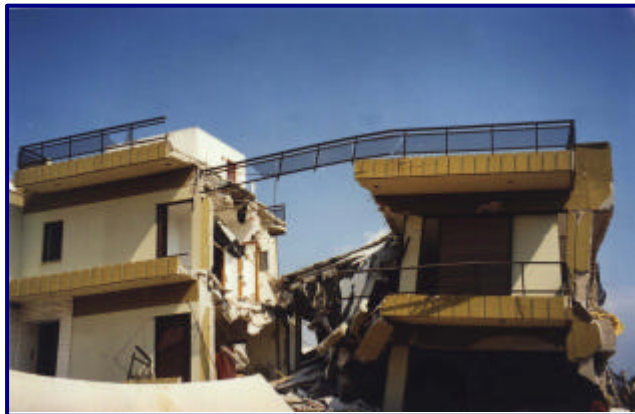
7 b . Partial collapse of the load bearing system
