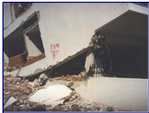
6. Collapse due to failure of columns at the soft ground floor
