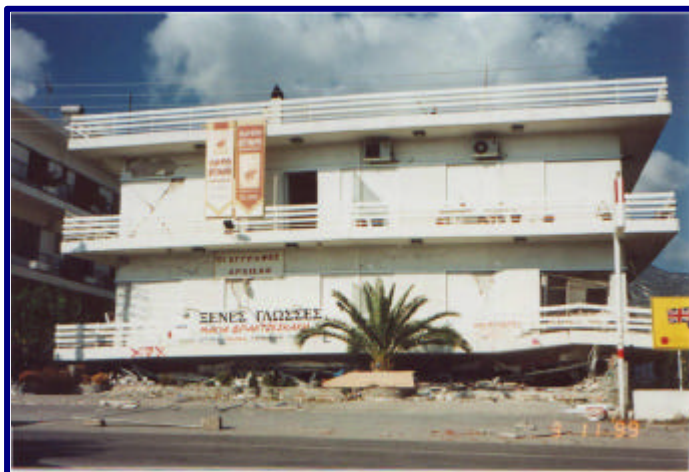
6. Collapse due to failure of columns at the soft ground floor
